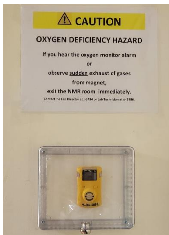
Oxygen monitor, Single Gas Clip, Model BW See Appendix B for its maintenance.
