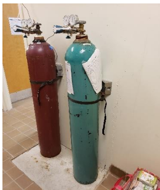
Cylinders secured to a wall.
