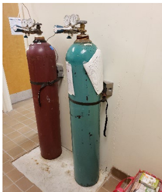
Cylinders secured to a wall.
